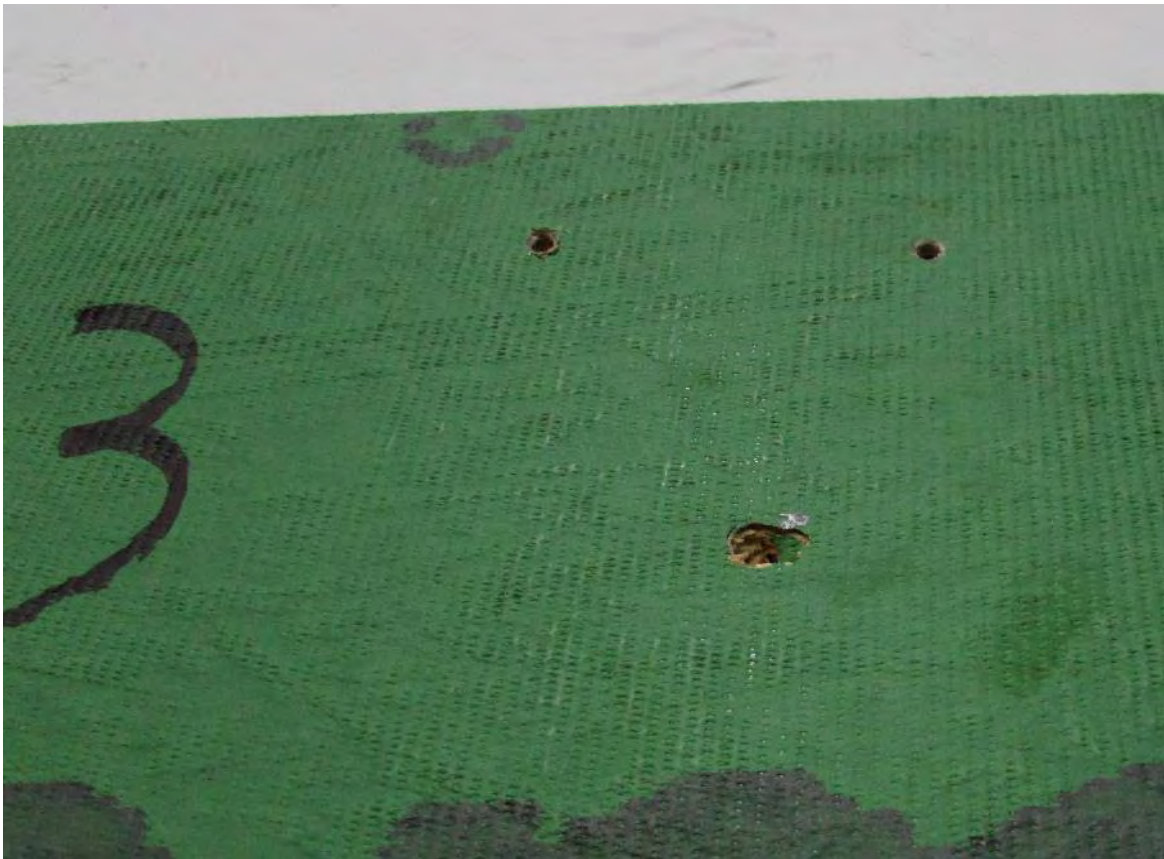
Sample 3 Failure (Sheathing Pull-over Pin Head)
