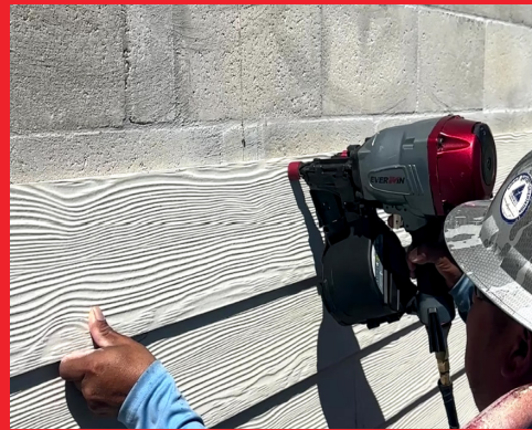
Cement Fiber Siding to Block
