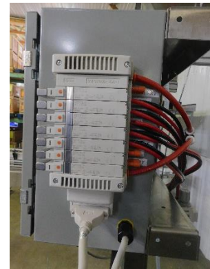
Figure 5-5 Air Solenoids
