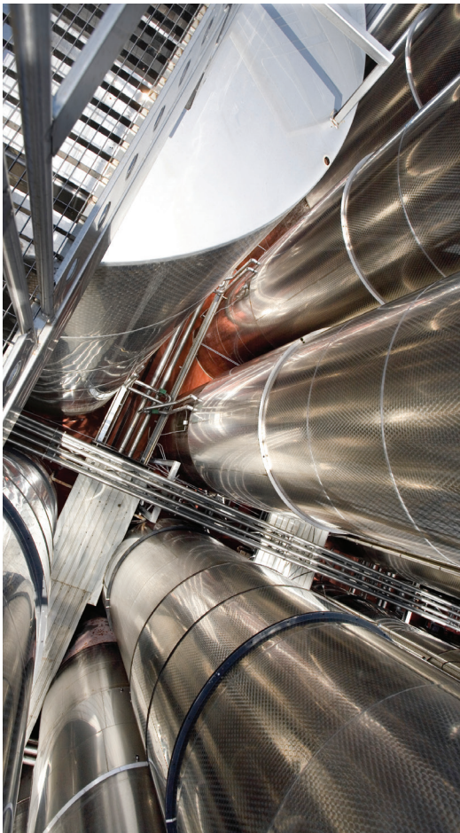
Silo, Tank and Hopper
