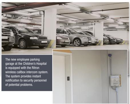
The system is very similar to the one already in place in the patient parking garage. A single callbox is installed in the center of each floor, near the stairs and elevator. A total of 8 callboxes are in-service in the employee garage. The callboxes communicate campus-wide, utilizing the 40-watt repeater and 50-foot antenna mounted on the hospital's roof.
