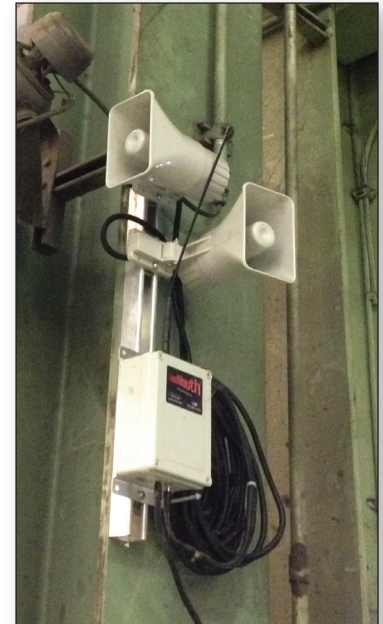
Two speakers connected to a single receiver provide maximum coverage from a single point.
