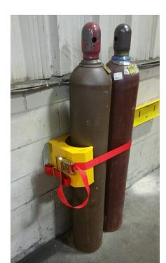
Also for use in storage of cylinders in stationary (wall mount) Industrial and Medical Facility's daily use or storage. Fasteners and spacers for wall mounting included.
